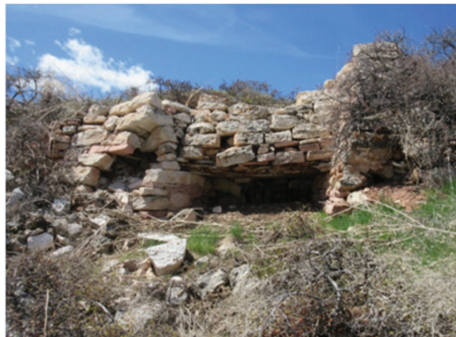
A more recent photo of the kiln around 2020 shows increased deterioration.
