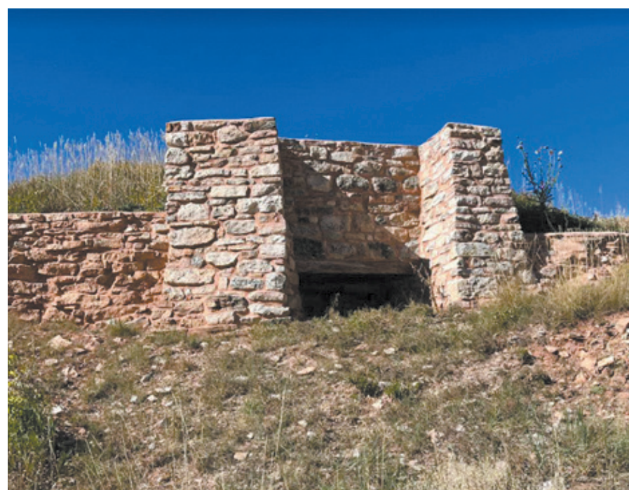
Restoration of the kiln brought it back to its 1979 appearance.
