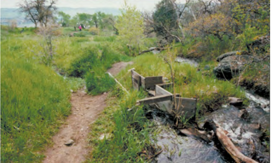
John C. Shaffer built a wooden diverter structure along Massey Draw and a ditch, aptly named Shaffer Ditch, to channel water to the Tinker Shaffer Reservoir. Work to restore the diverter is slated to begin later this year.
